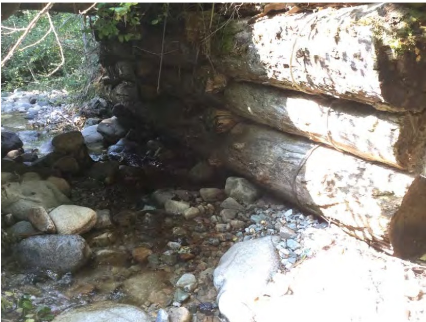
Right Bank Abutment when facing downstream
