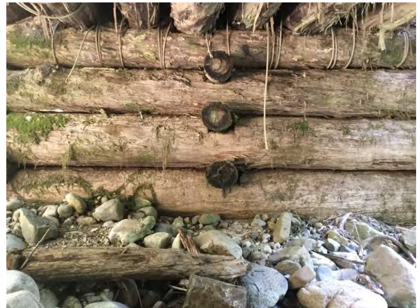
Left Bank Abutment when facing downstream
