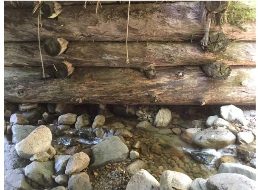
Right Bank Abutment when facing downstream
